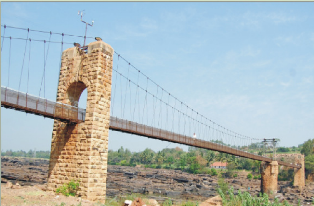
Hanging Bridge for workmento cross during monsoon ←
